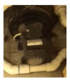
3. Install Variable Speed Drives on the main circulation pumps, We would recommend using a swimming pool specialist as they need to consider the flow switch in the Automatic Dosing Unit.
